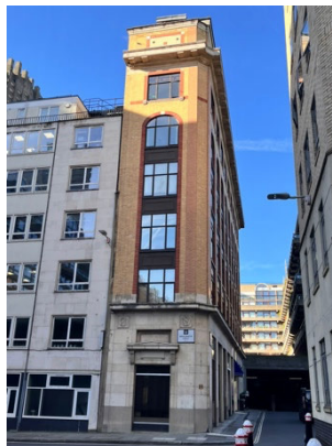
Bridgewater House eastern elevation
