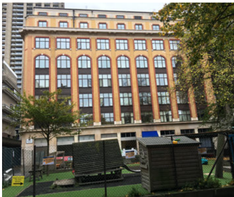
Bridgewater House northern elevation
